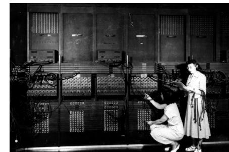
A small amount of time is required in preparing the ENIAC for a problem by such steps as setting program switches, putting numbers into the function table memory by setting its switches, and establishing connections between units of the ENIAC for the communication of programming and numerical information.
